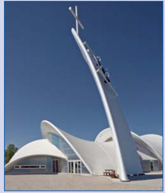
Front view of church
