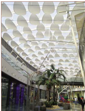
Interior views, with additional membrane shading (IASO, S.A.)
